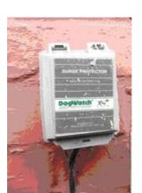
usually on the outside wall of the building in which the transmitter is located. Open the surge protector by lifting the flap upwards, inside there is three copper screws; Place a screwdriver or coin
