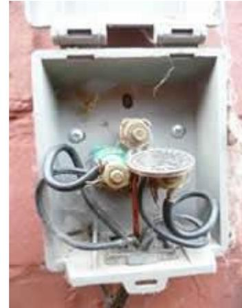
Please note if you have a beeping noise before carrying out this test and the green light is not showing on the transmitter this test will confirm that your cable is broken – when placing the bridge across the surge protector the green light should illuminate and the beeping should stop (a loop has been formed between the transmitter and the surge protector – when you remove the coin the beeping will start again as the loop has been broken).
